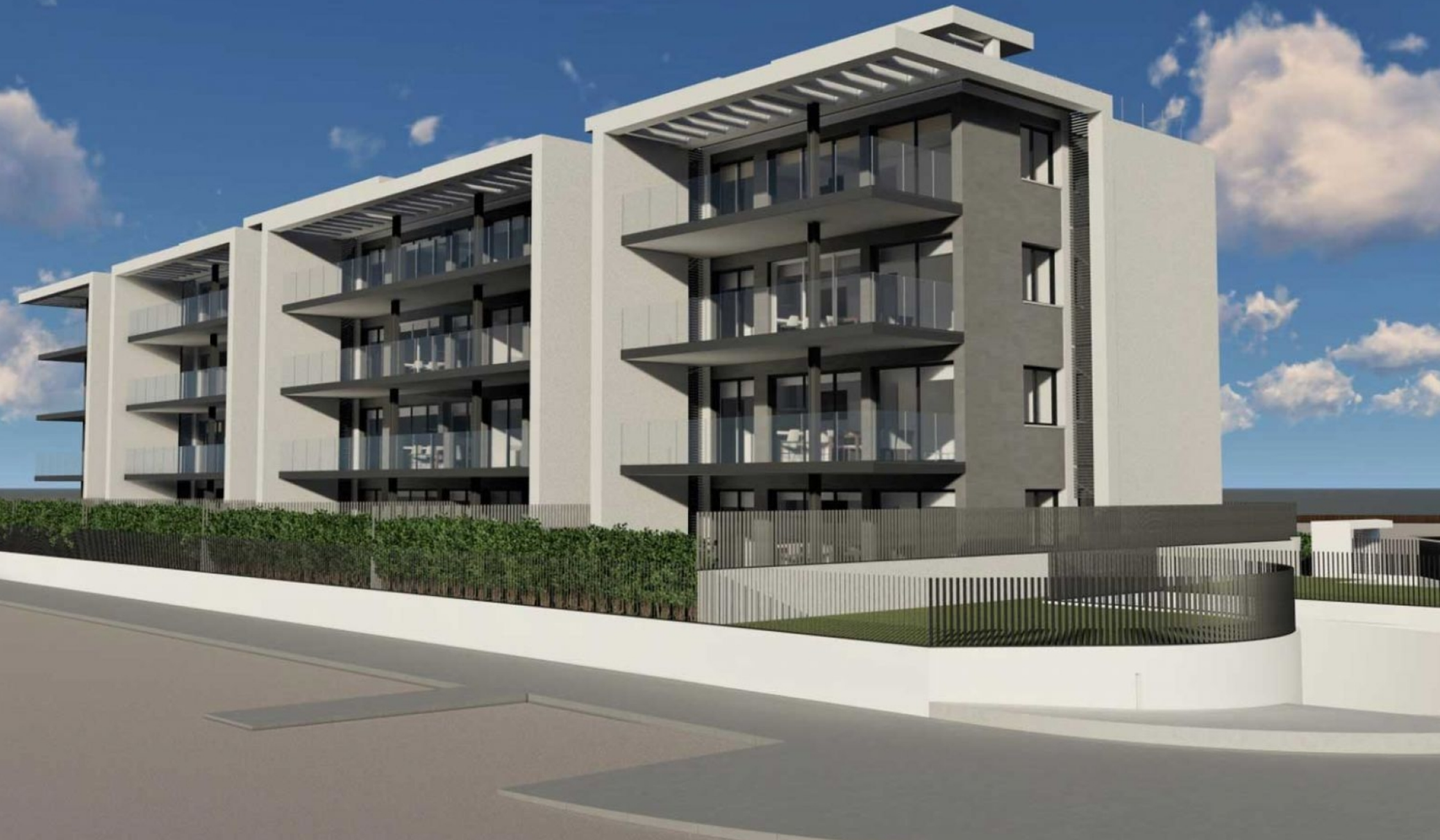
New construction ground floor under construction on the arenal beach of Jávea MONTAÑAR - EL ARENAL, JÁVEA/XÀBIA - REF. A0-A
