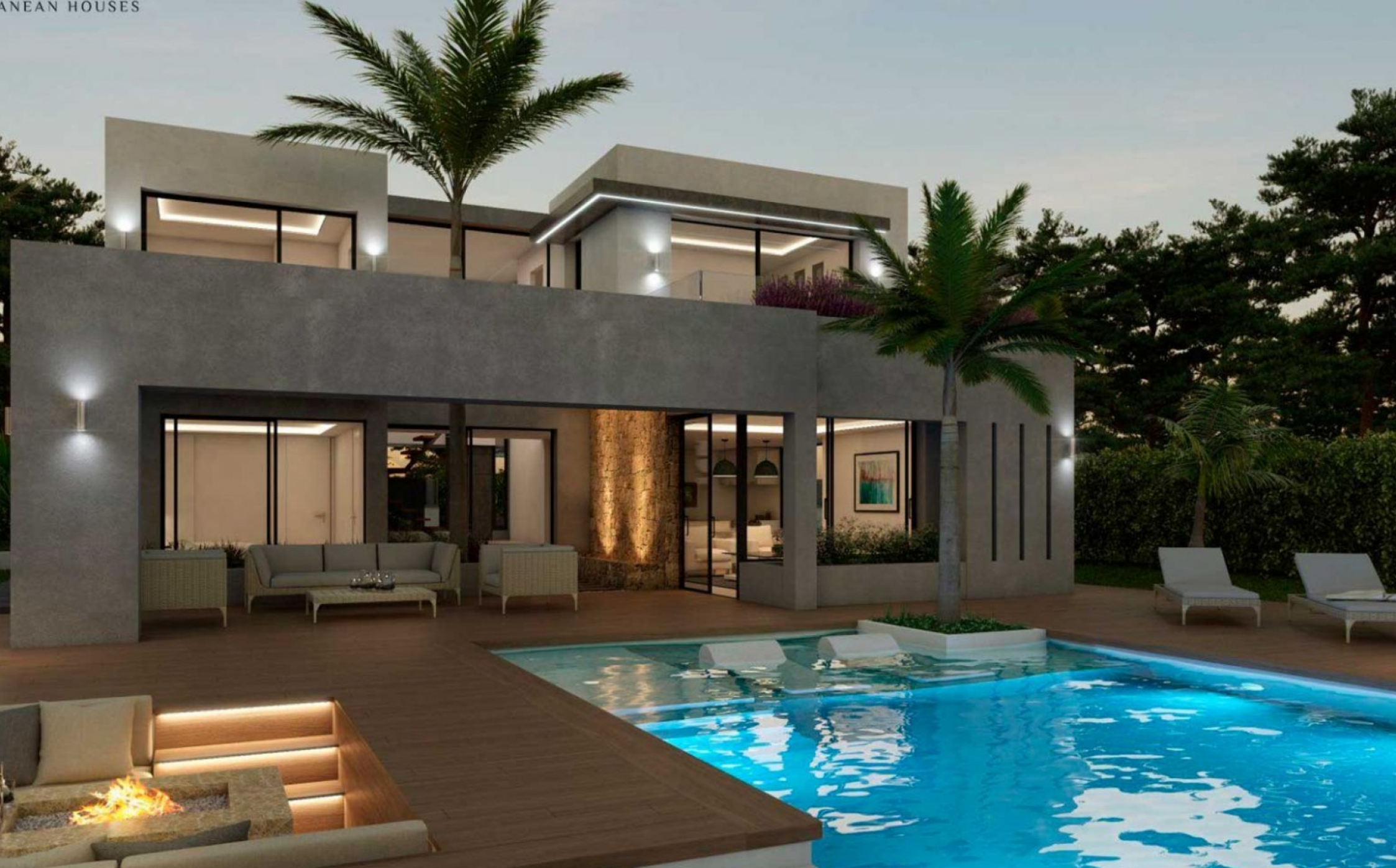
Newly built villa under construction in La Guardia BALCÓN AL MAR - PORTICHOL, JÁVEA/XÀBIA - REF. V-141
