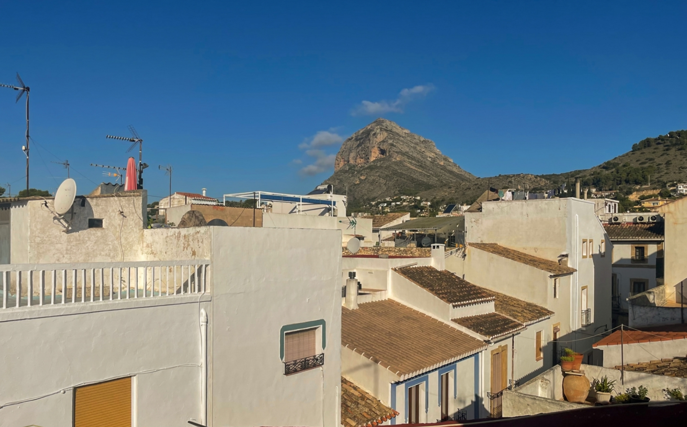
Townhouse to renovate in Jávea OLD TOWN CENTER, JÁVEA/XÀBIA - REF. V-310
